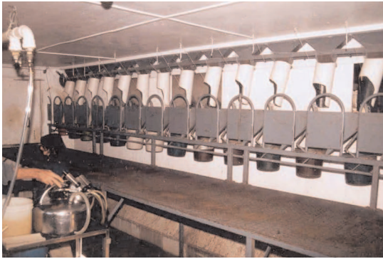
One x 12 cascading yokes and elevated platform.
