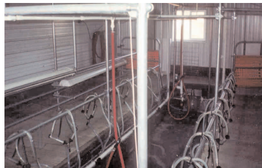
Two x 16 crowding system low line pipeline (Kieffer, Wisconsin).
